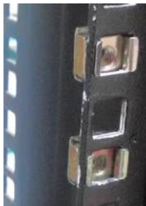
5. Install the rack assembly brackets onto the rack by using two screws. It is
